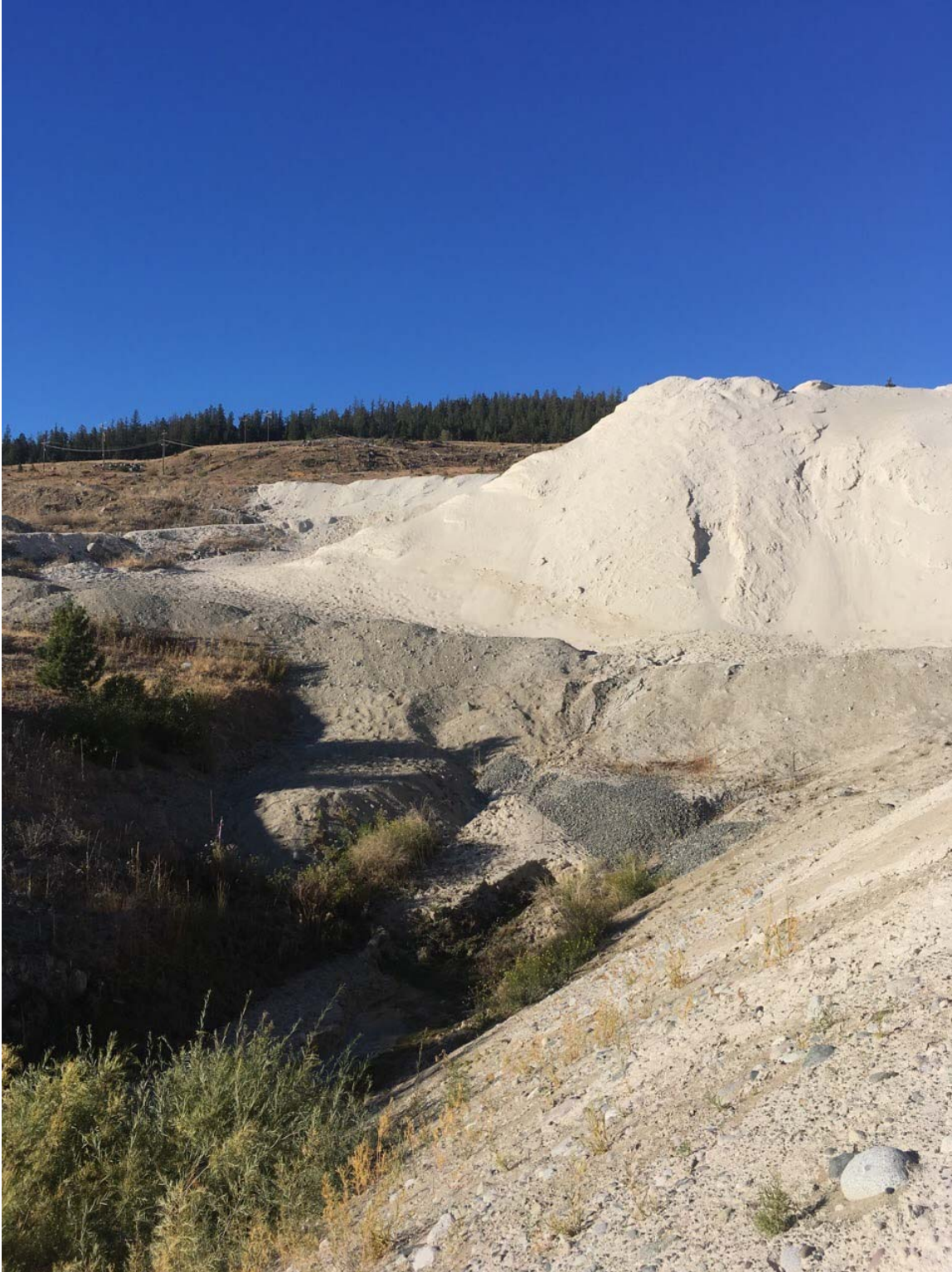
Photo II-A-14 North Dam Drain – Facing North (LL-2017-16)
