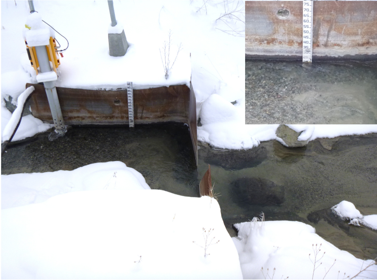
Photo 7 – Point B weir with accumulated sediment in weir box and outfall.
