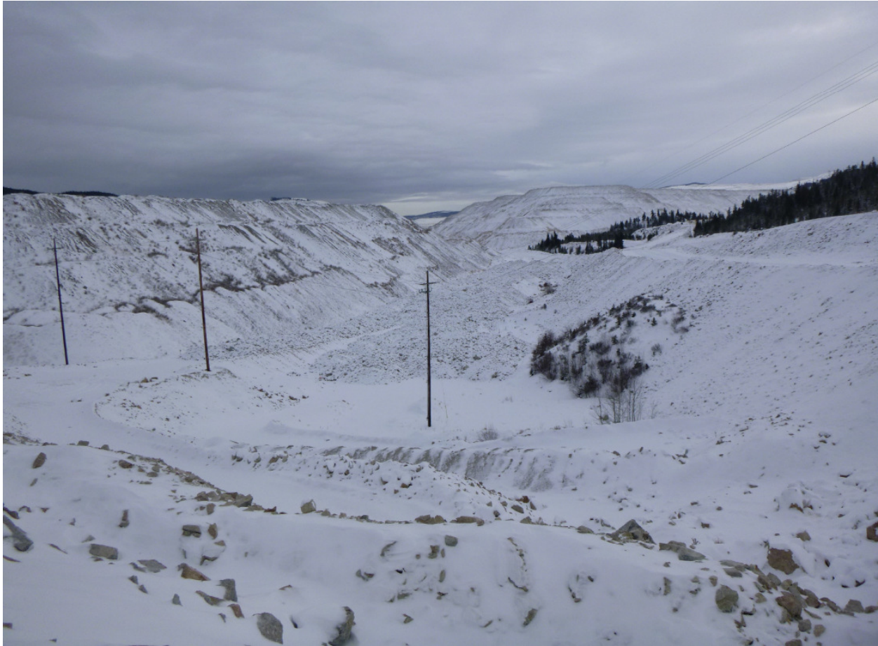
Photo 4 – Recently dumped d/s RF2 material observed between west side of I-9 waste dump and the west access road on the dam (looking southeast).
