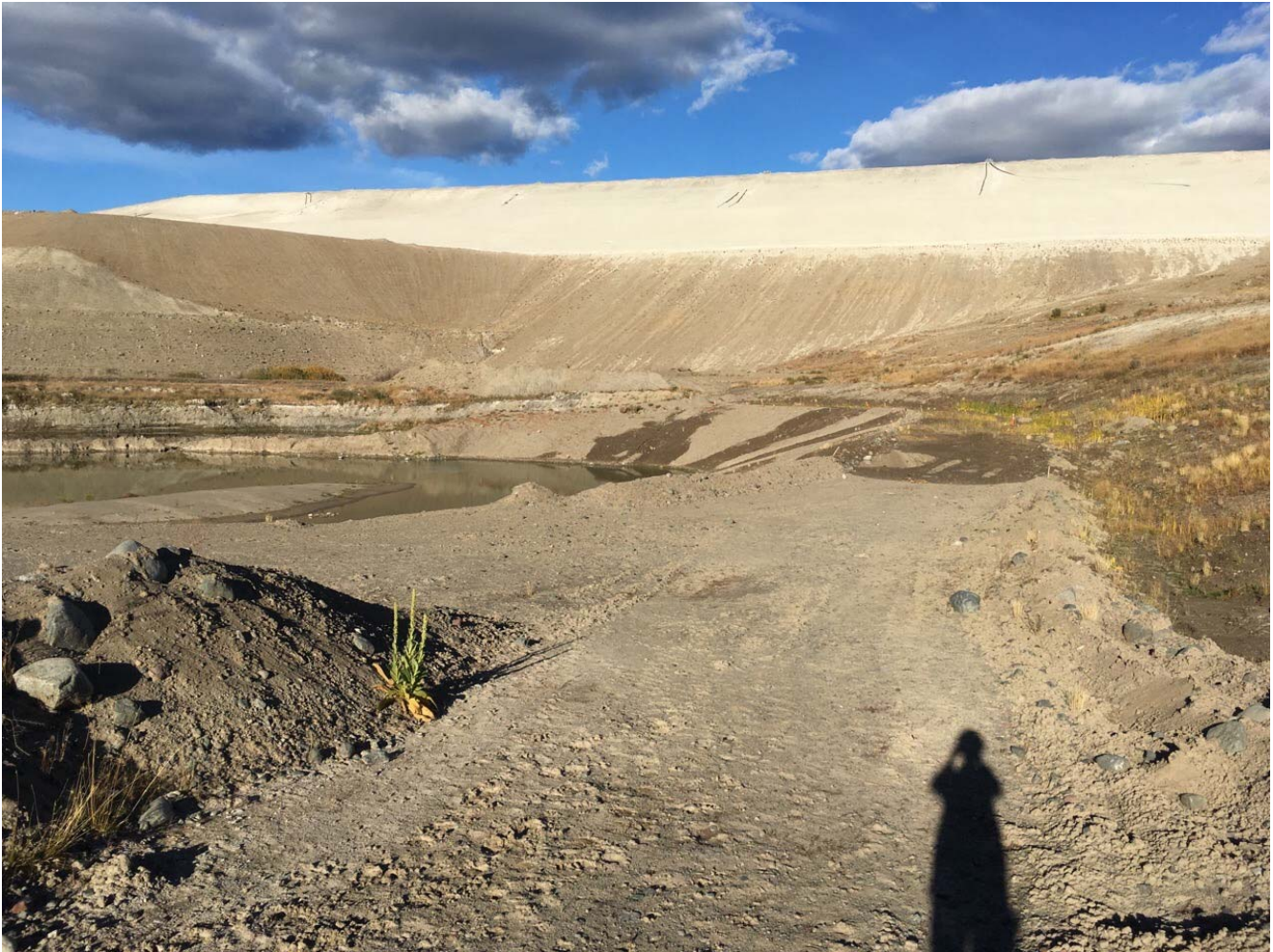
Photo II-C-17 Slimes Pond 3 (partially constructed) – Ponded Water on Crest from Spring Lines in Slope – Facing East (SS-2017-11)
