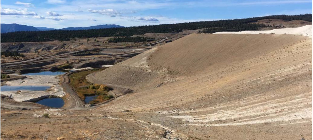
Photo II-A-18 Toe and Downstream Face of South Dam - Facing Northwest (LL-2017-24)
