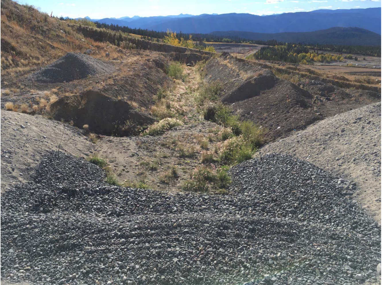
Photo II-A-10 South Dam – Major Drain Outlet with <1 L/min Flow Rate (LL-2017-05)
