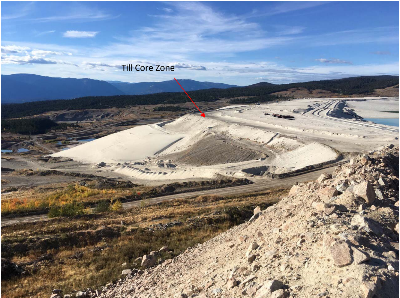
Photo II-A-8 Downstream face at South Abutment - Facing North (LL-2017-02)
