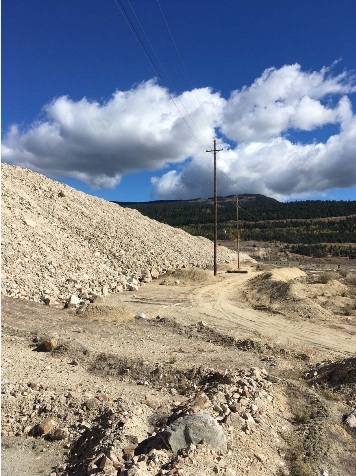
Photo II-B-10 Downstream Face of Dam - Facing Northeast (HH-2017-15)
