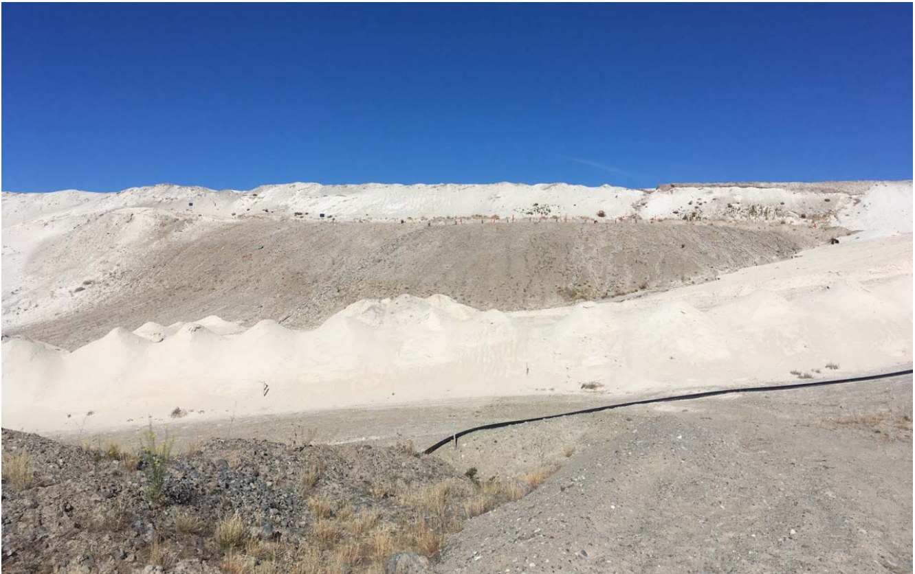
Photo II-A-21 Downstream Slope at South Abutment - Facing Northwest (LL-2017-03)
