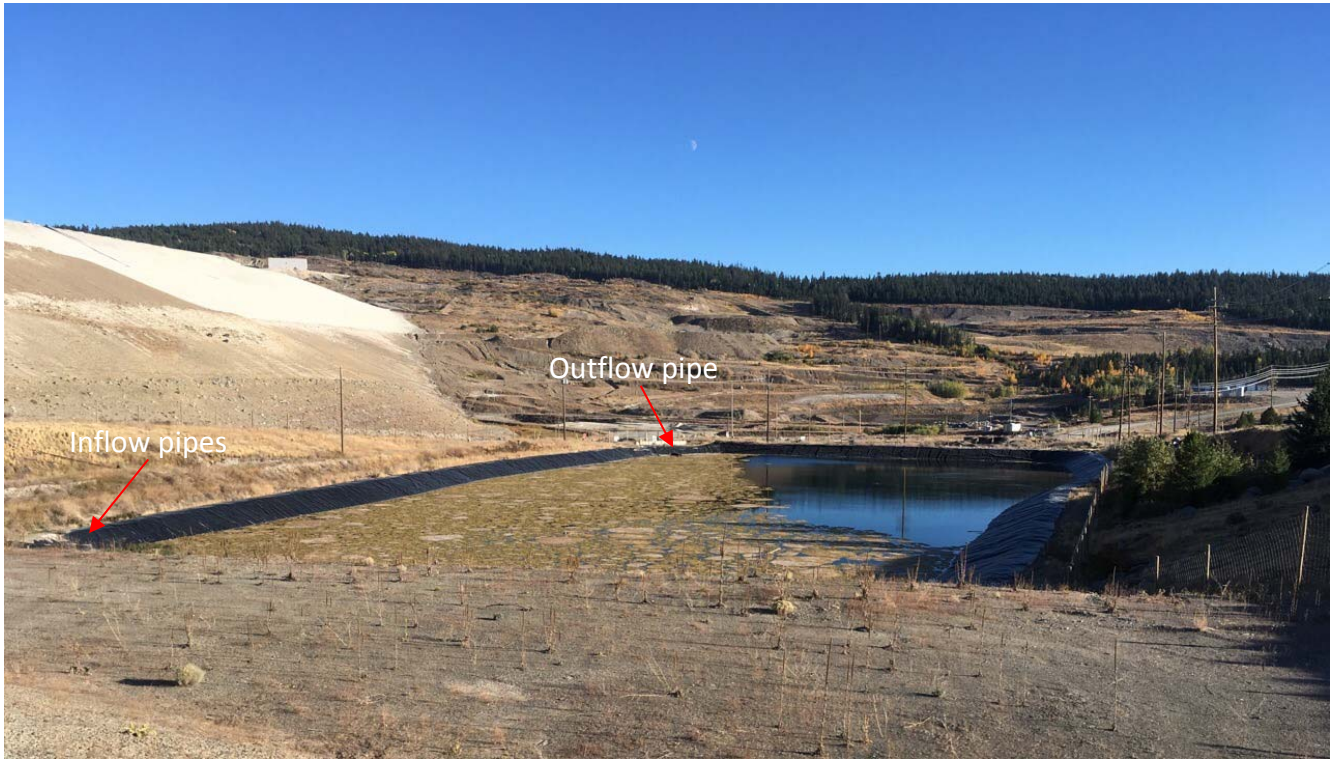
Photo II-C-9 Seepage Pond 2 Overview – Facing Southeast (SS-2017-06)
