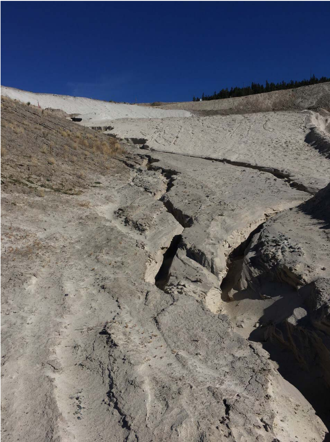
Photo II-A-9 South Dam – Erosion from Cyclone House Spill (LL-2017-06)
