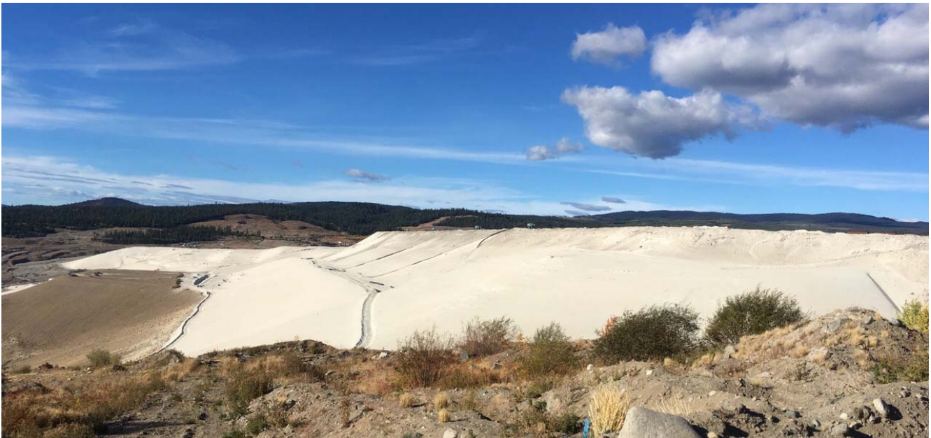
Photo II-A-19 Downstream Slope of South Dam - Facing North (LL-2017-04)
