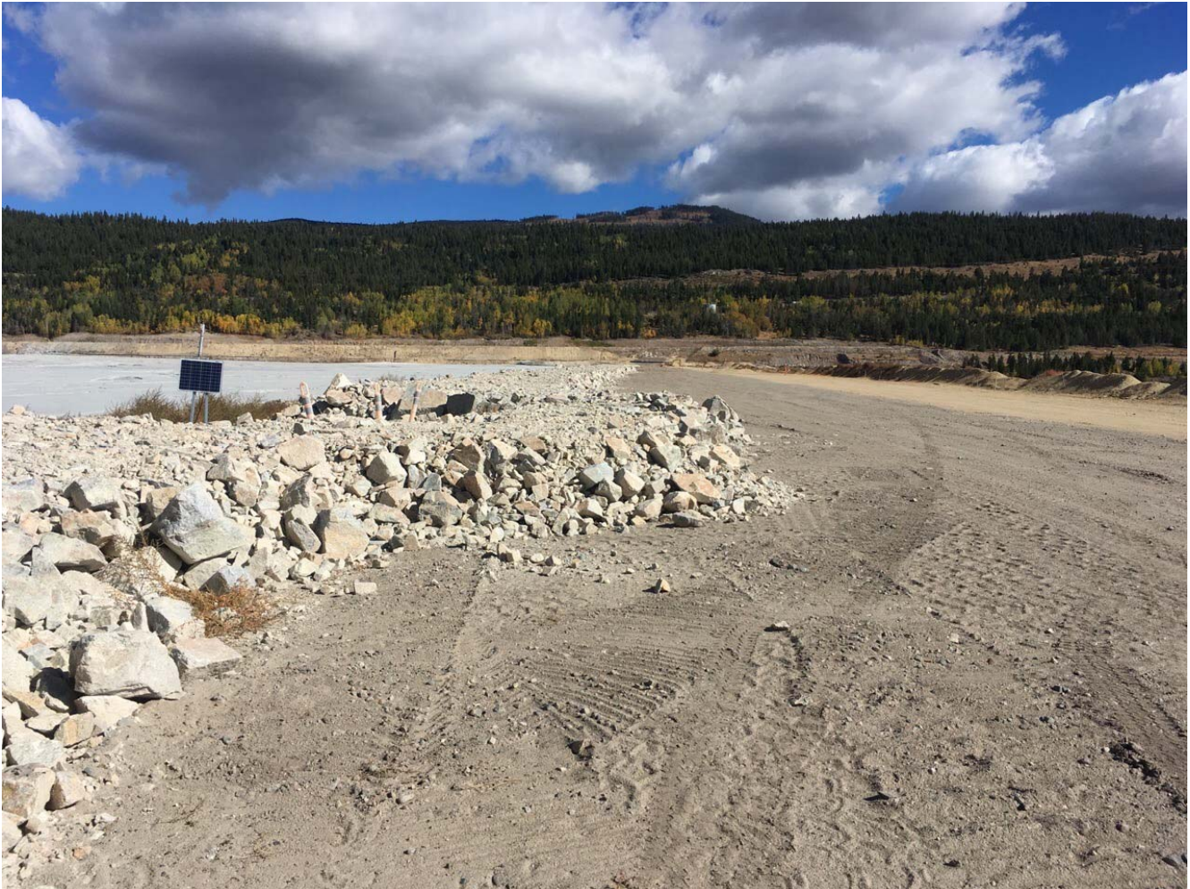
Photo II-B-4 Till Core Zone - Facing Northeast; upstream buffer at HHVWP15-22; RF2 material has been placed on Till Core Zone (HH-2017-06)
