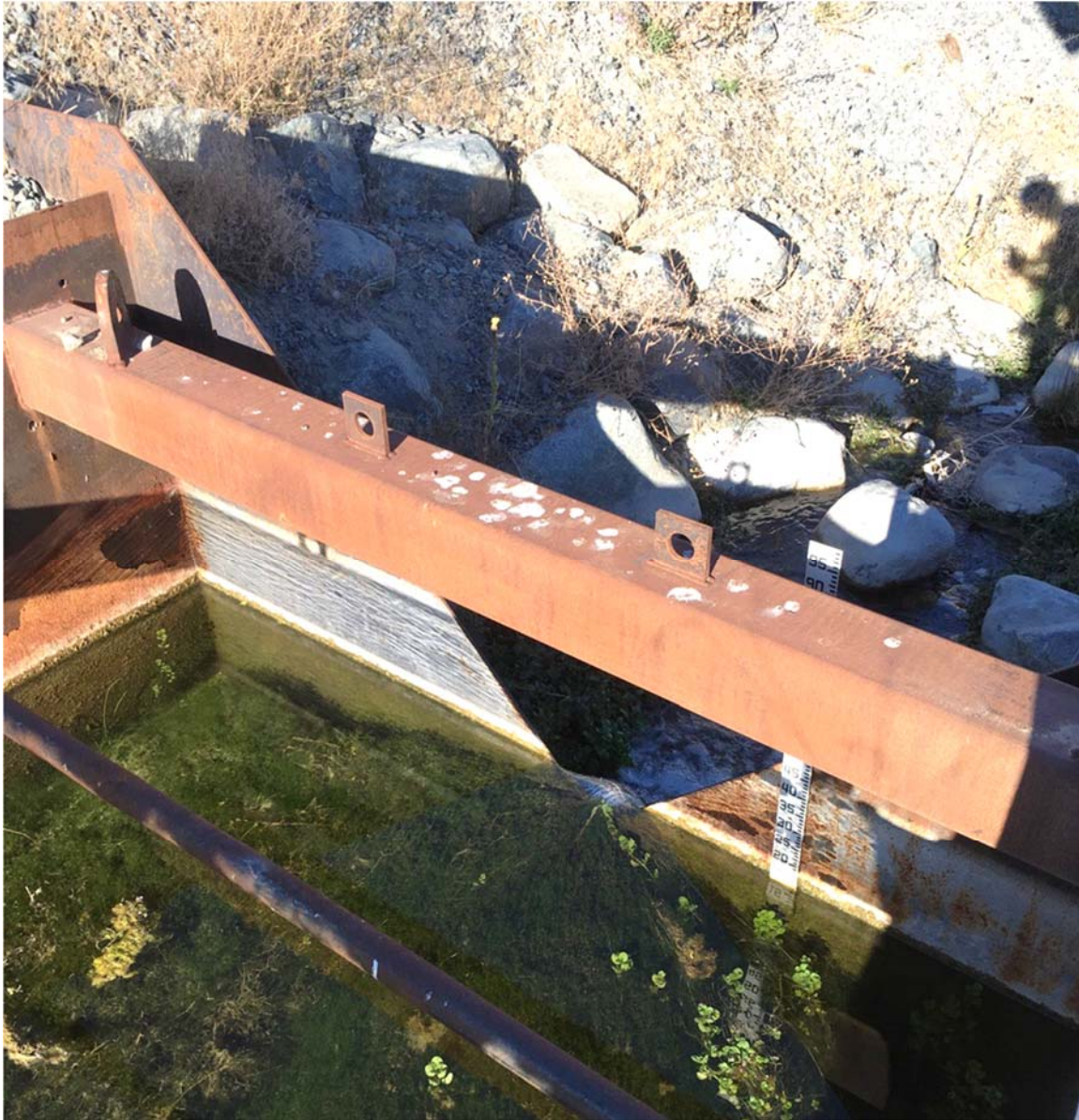
Photo II-A-25 Seepage Pond 2 Weir (LL—FS-04) (LL-2017-21)
