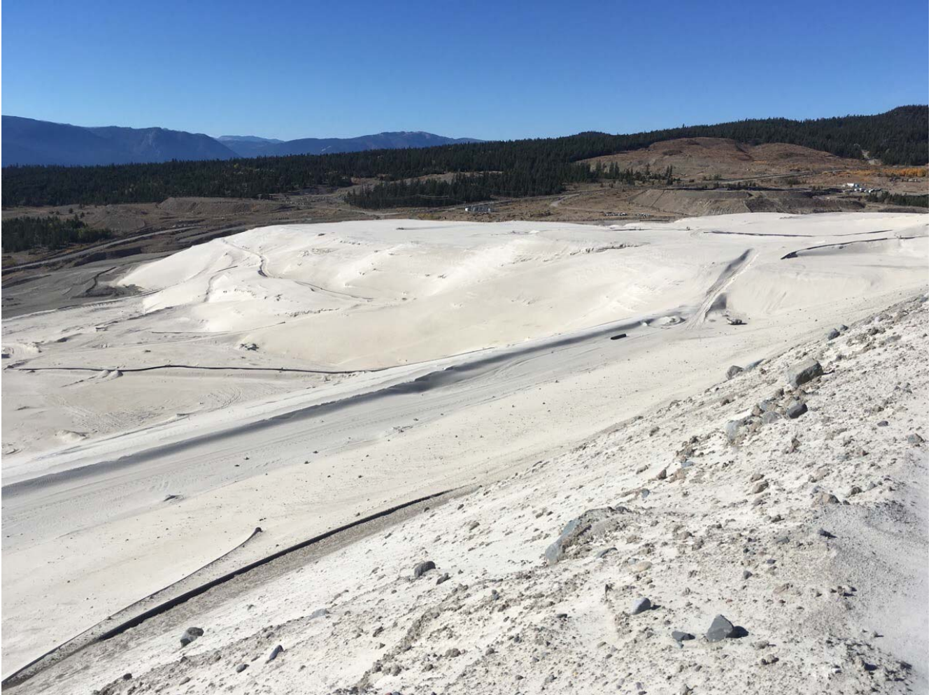
Photo II-A-17 North Buttress Berm South Slope – Facing Northwest (LL-2017-19)
