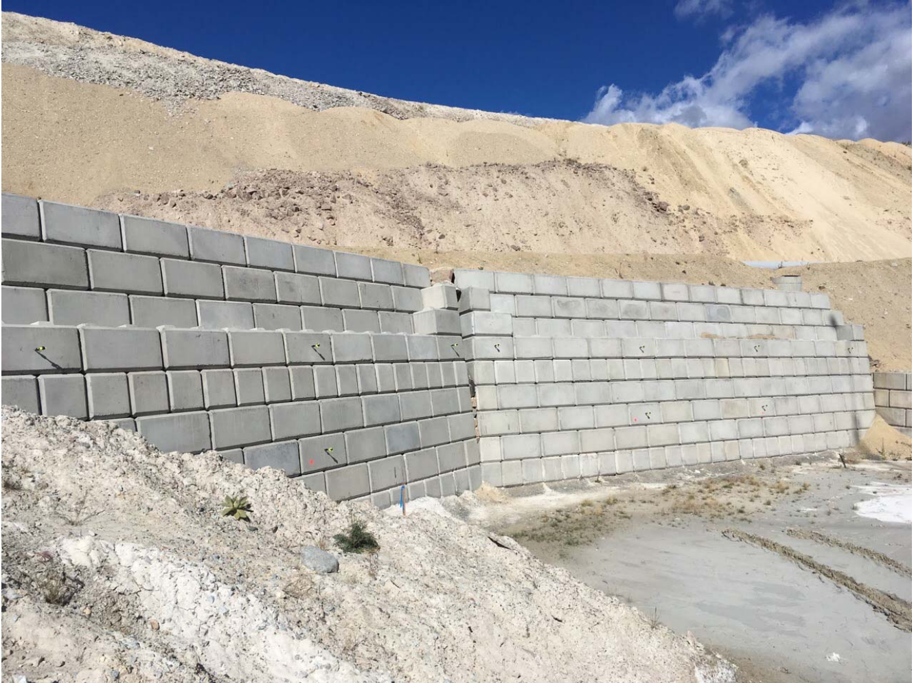
Photo II-B-15 Lock-block Retaining Wall at Toe of Dam; new survey prisms (HH-2017-11)
