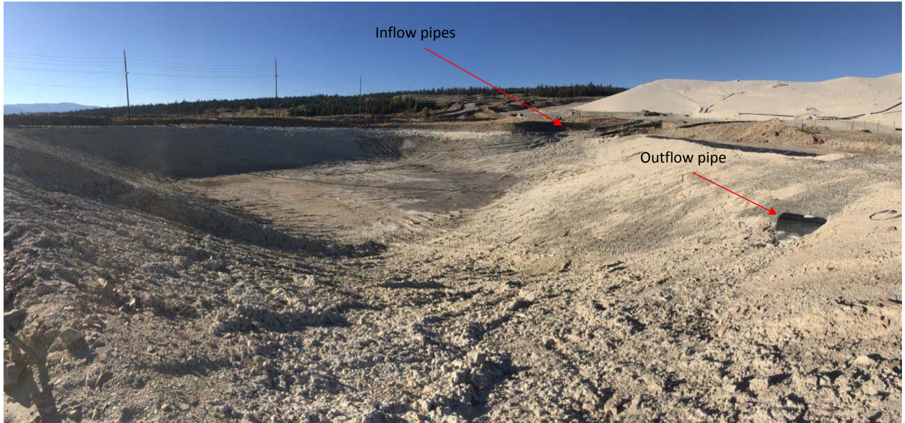
Photo II-C-6 Slimes Pond 2 – Slimes excavate/removed in 2017 – Facing North (SS-2017-05)
