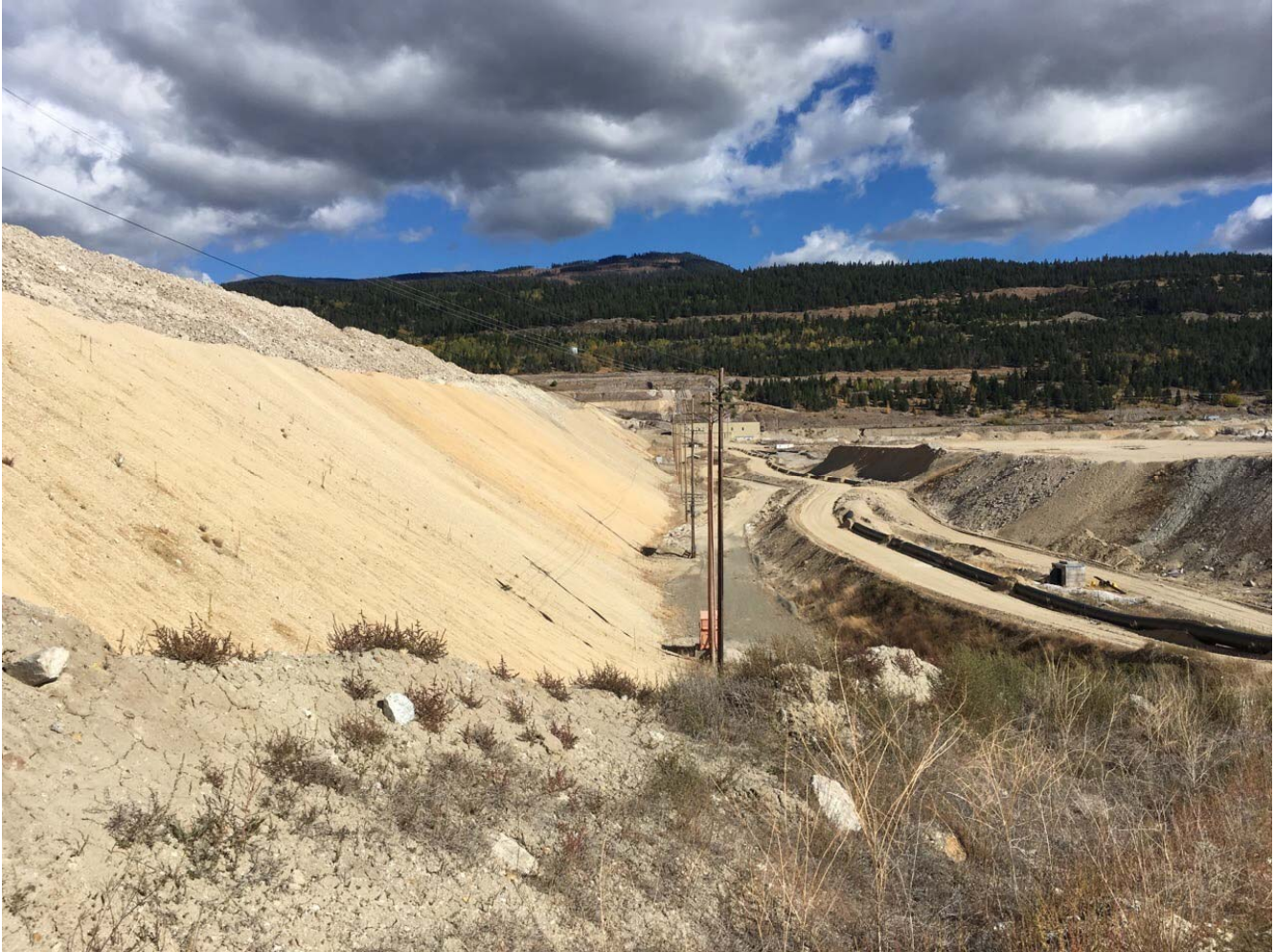
Photo II-B-11 Downstream Toe of Dam - Facing Northeast (HH-2017-14)
