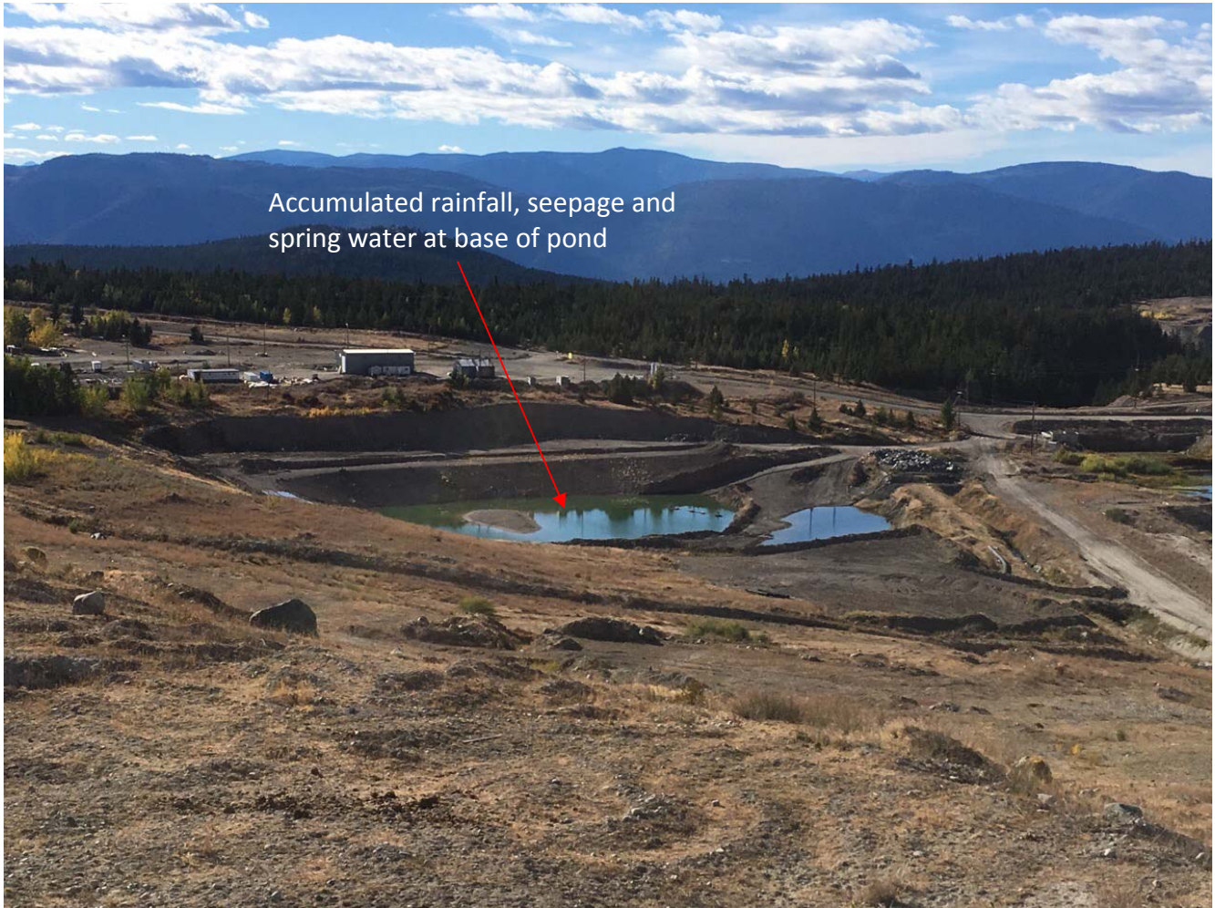
Photo II-C-15 Slimes Pond 3 (partially constructed) – Facing West (SS-2017-01)
