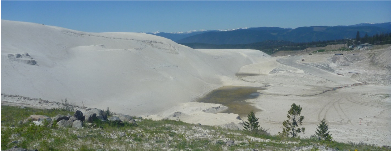
Photo 1- Poned Water At North Toe of North Buttress Berm (facing west)
