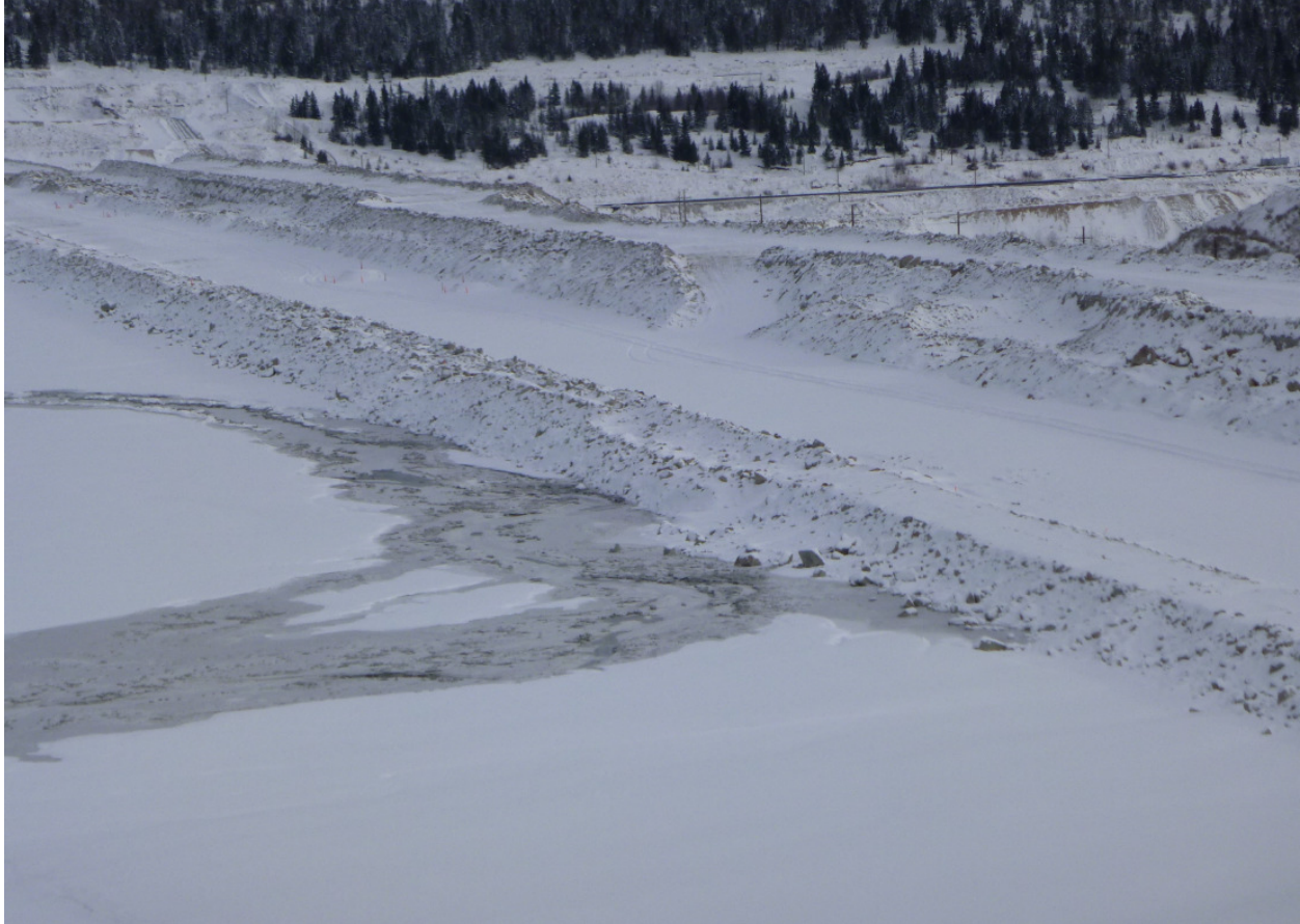
Photo 3 - Evidence of recent discharge from SS1/SS2 along/near the u/s RF2 face approximately between Sta. 0+600 to 0+750 (looking east).
