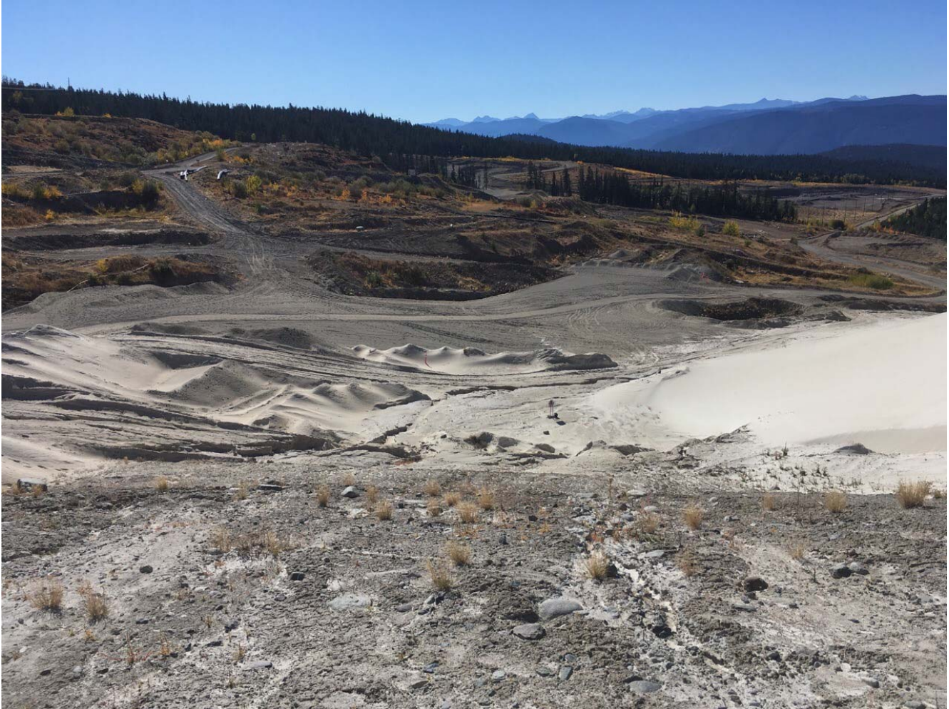
Photo II-A-20 Downstream Toe at South Abutment - Facing East (LL-2017-07)
