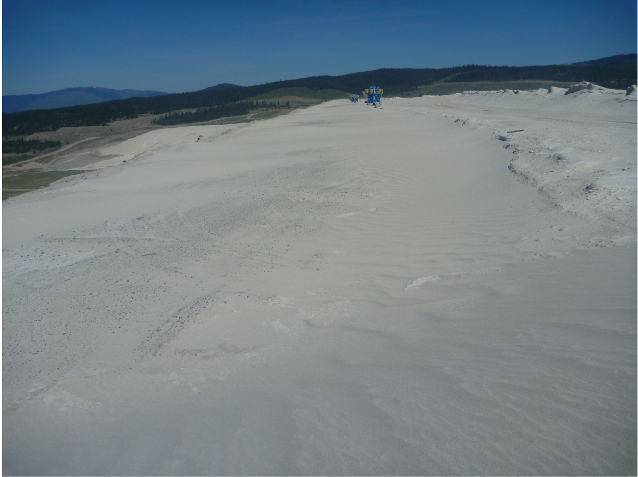
Photo 5 – Windblown sand cover on Till Core Zone
