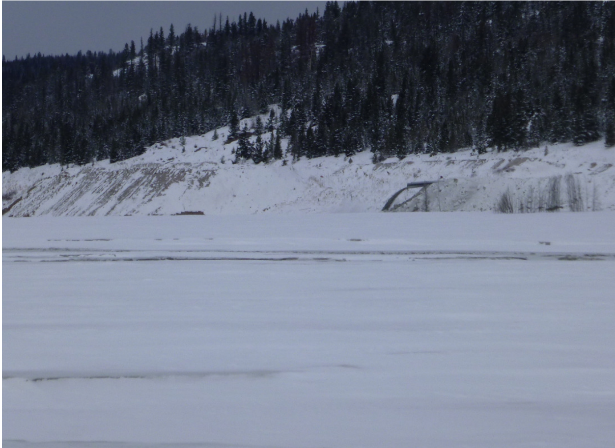
Photo 7 – Tailings discharging northwest of the east abutment (looking northeast).
