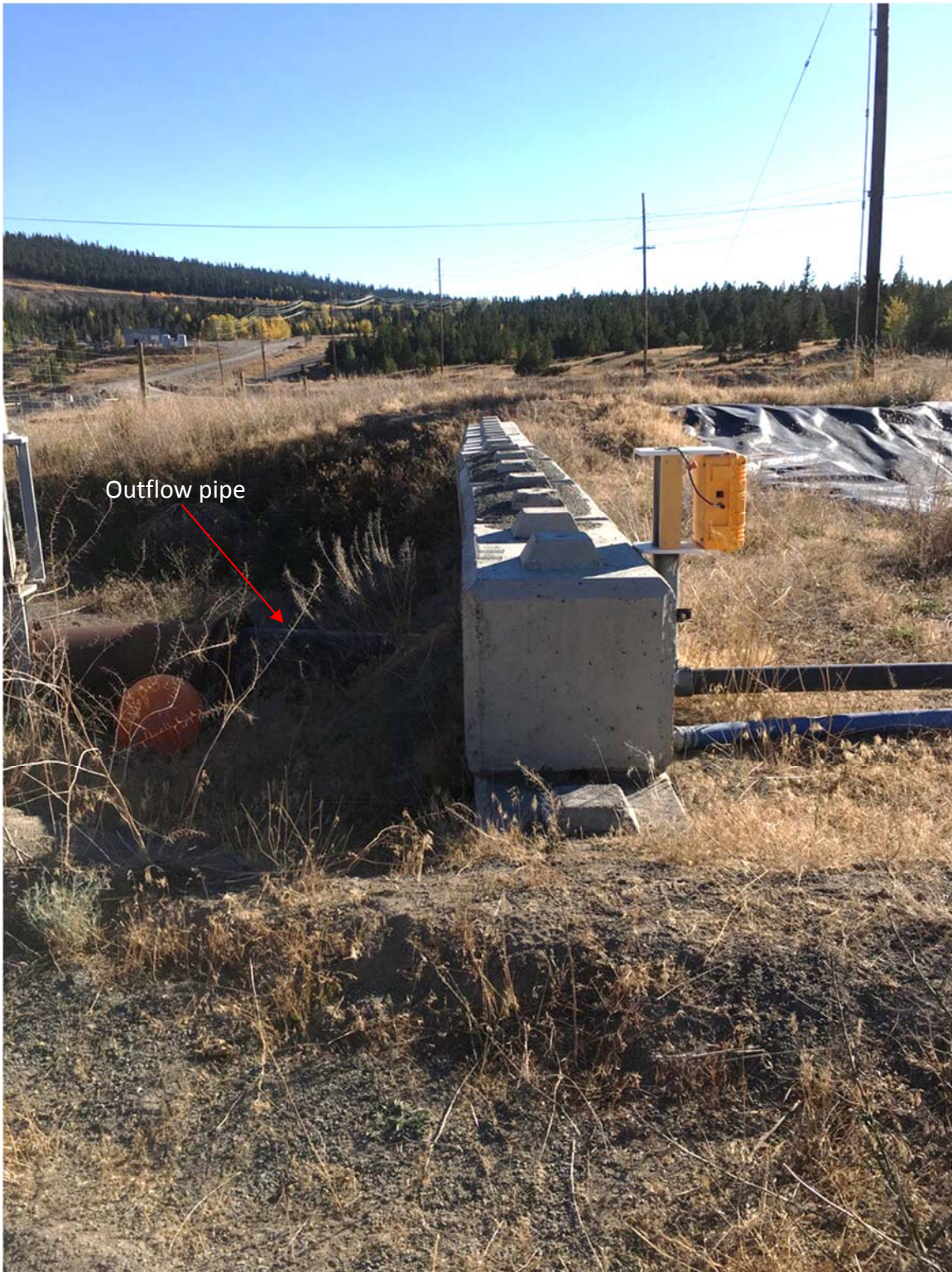
Photo II-C-12 Seepage Pond 2 Outlet Pipe and Lock-block Wall (SS-2017-07)
