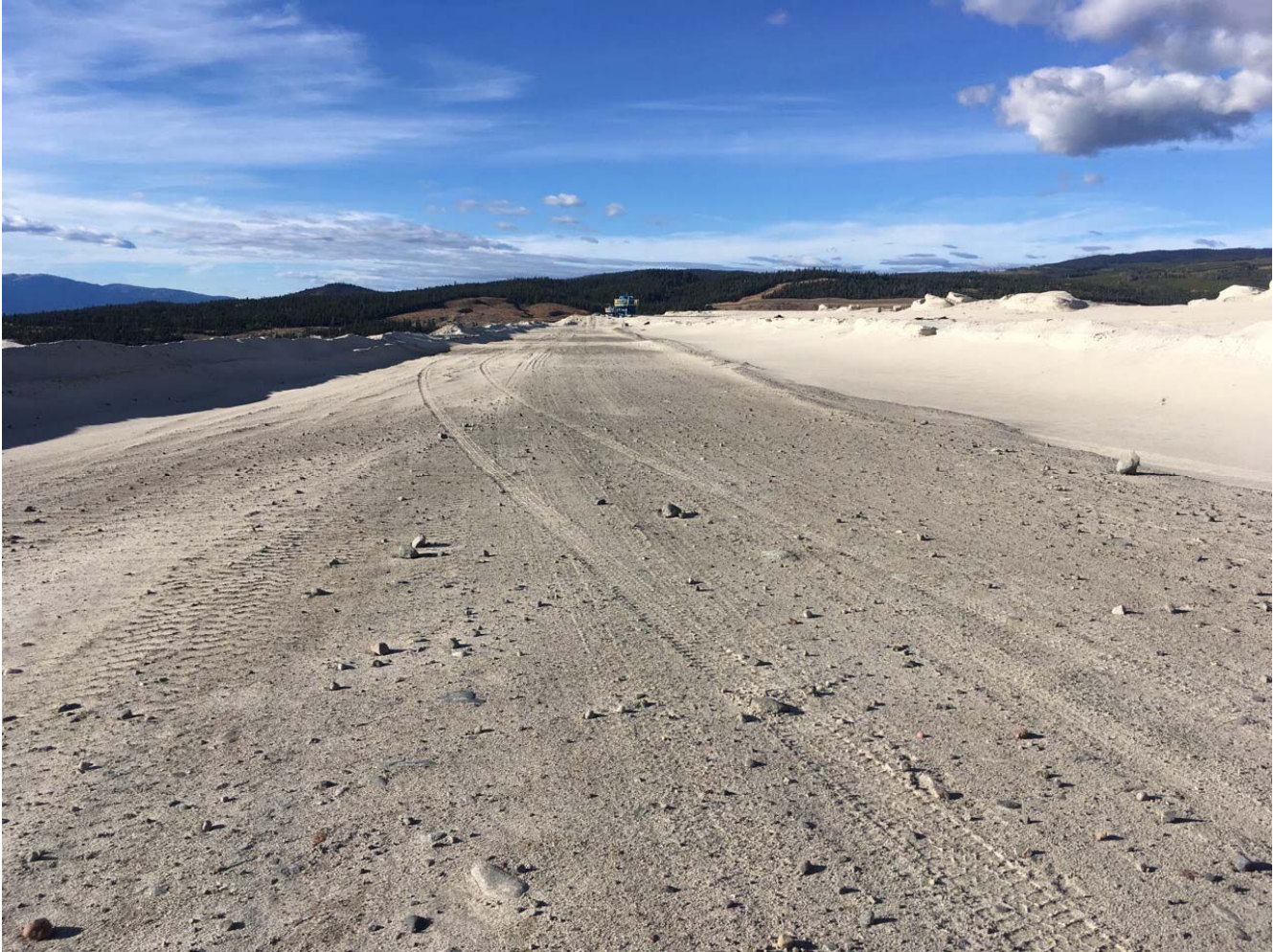
Photo II-A-11 South Dam Till Core Zone – Facing Northwest (LL-2017-08)
