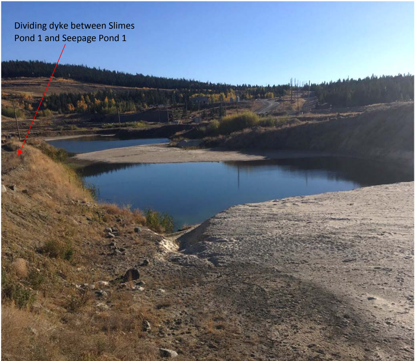
Photo II-C-2 Slimes Pond 1 – Facing South (SS-2017-04)
