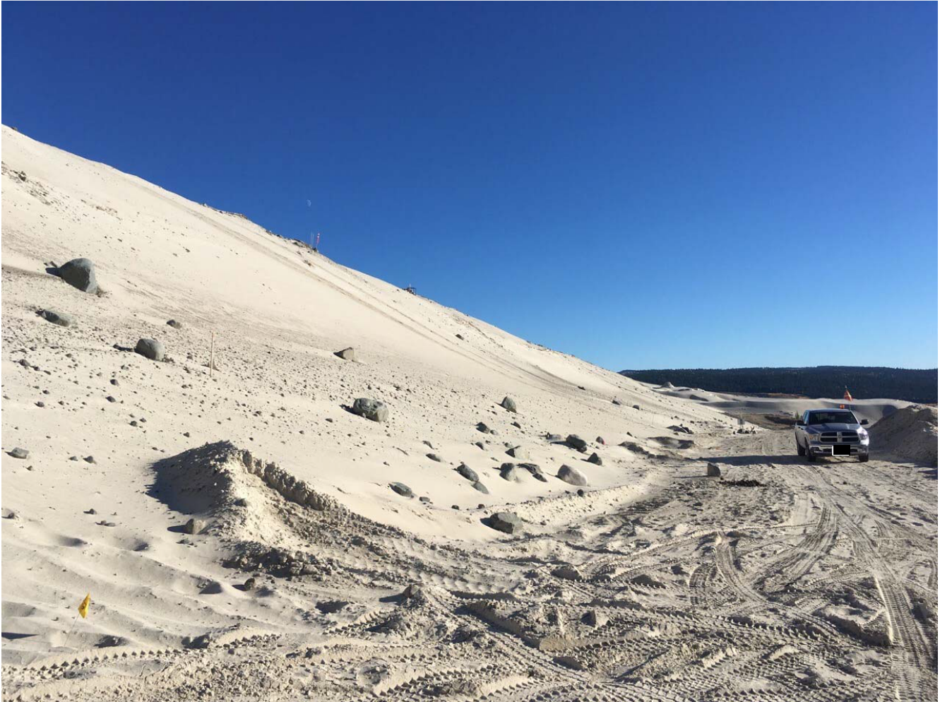
Photo II-A-13 North Dam Downstream Toe – Facing South (LL-2017-16)
