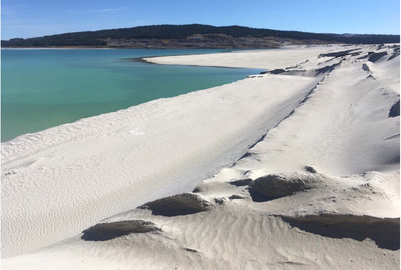
Photo II-A-4 Upstream Dam Face with Undercutting and Overhanging at Old Overflow Discharge Location – Facing East (LL-2017-13)
