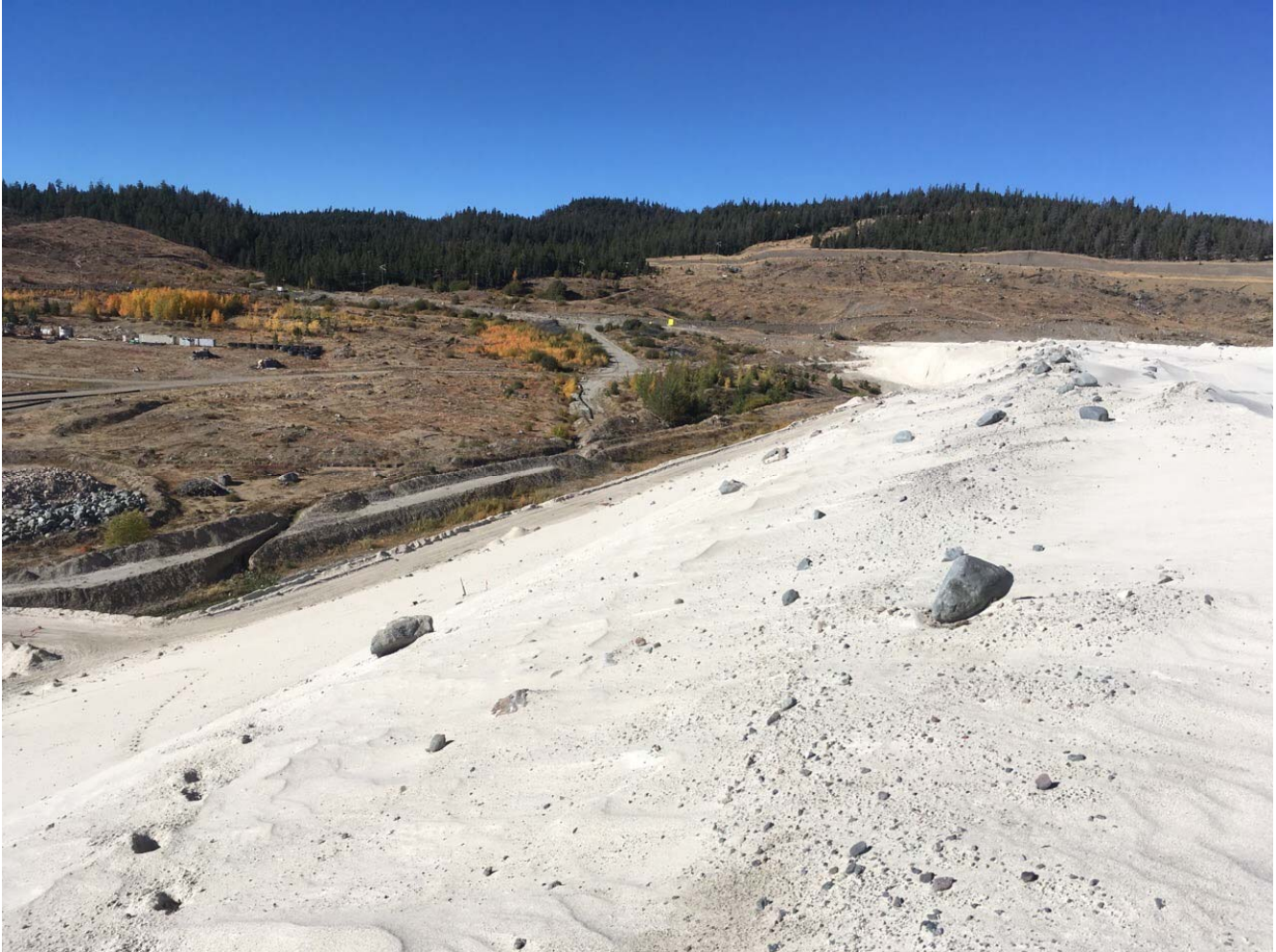
Photo II-A-15 North Dam Downstream Slope – Facing North (LL-2017-17)
