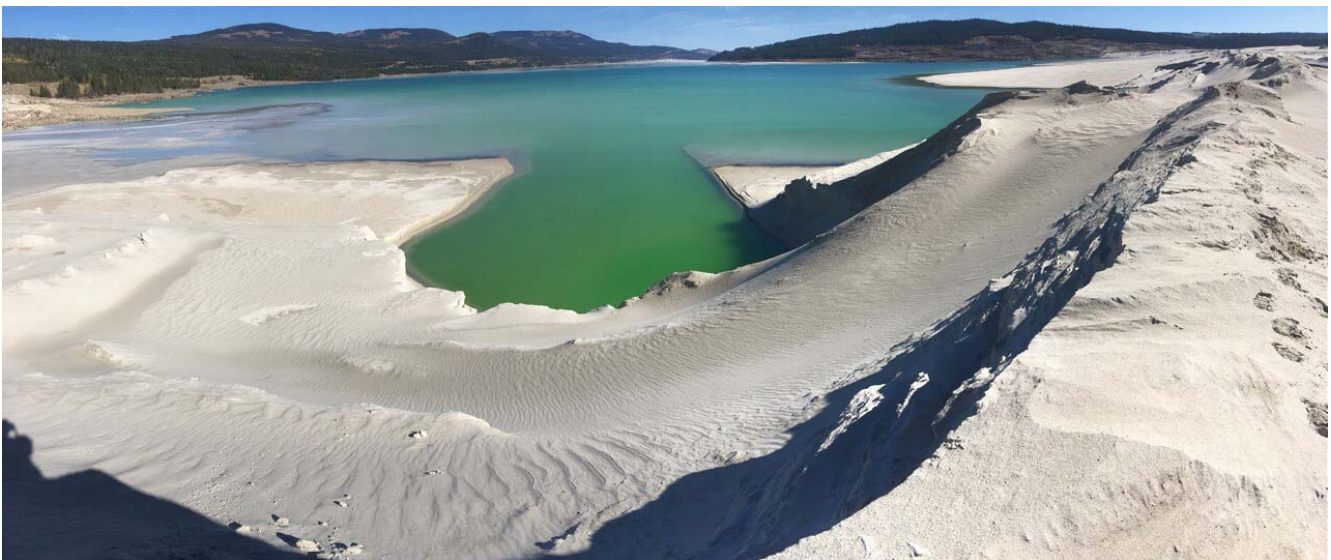
Photo II-A-4 Upstream Dam Face with Undercutting and Overhanging at Old Overflow Discharge Location – Facing East (LL-2017-13)
