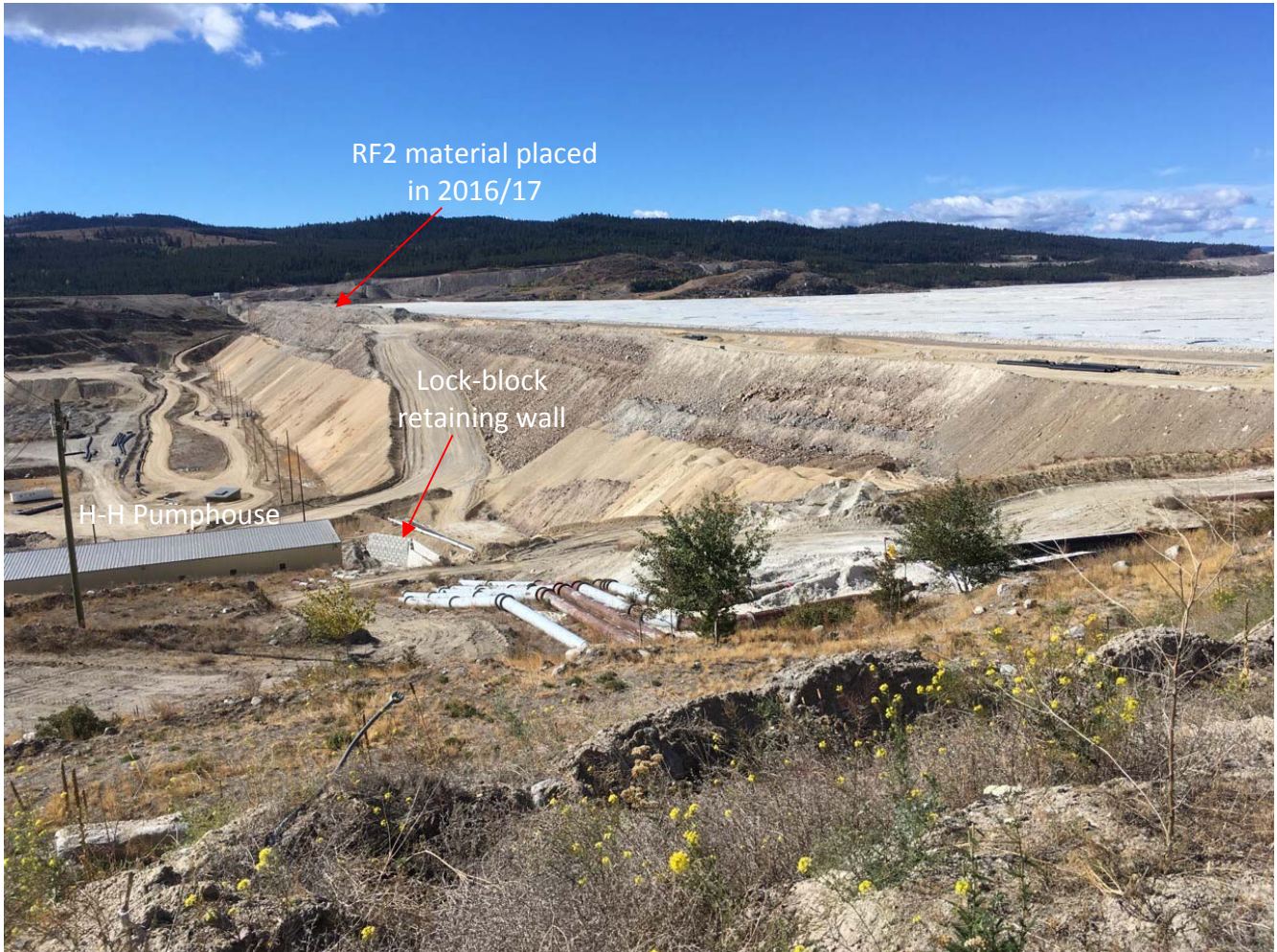
Photo II-B-14 Downstream Face of Dam - Facing West (HH-2017-10)
