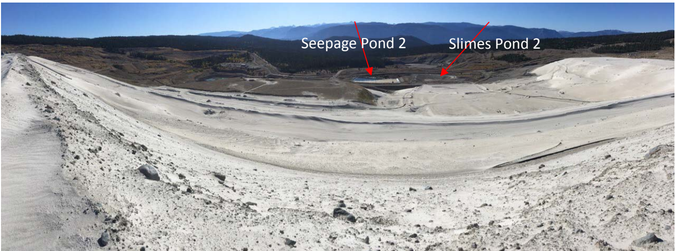
Photo II-A-22 Valley Buttress and Valley Buttress Berm Extension - Facing West (LL-2017-19)
