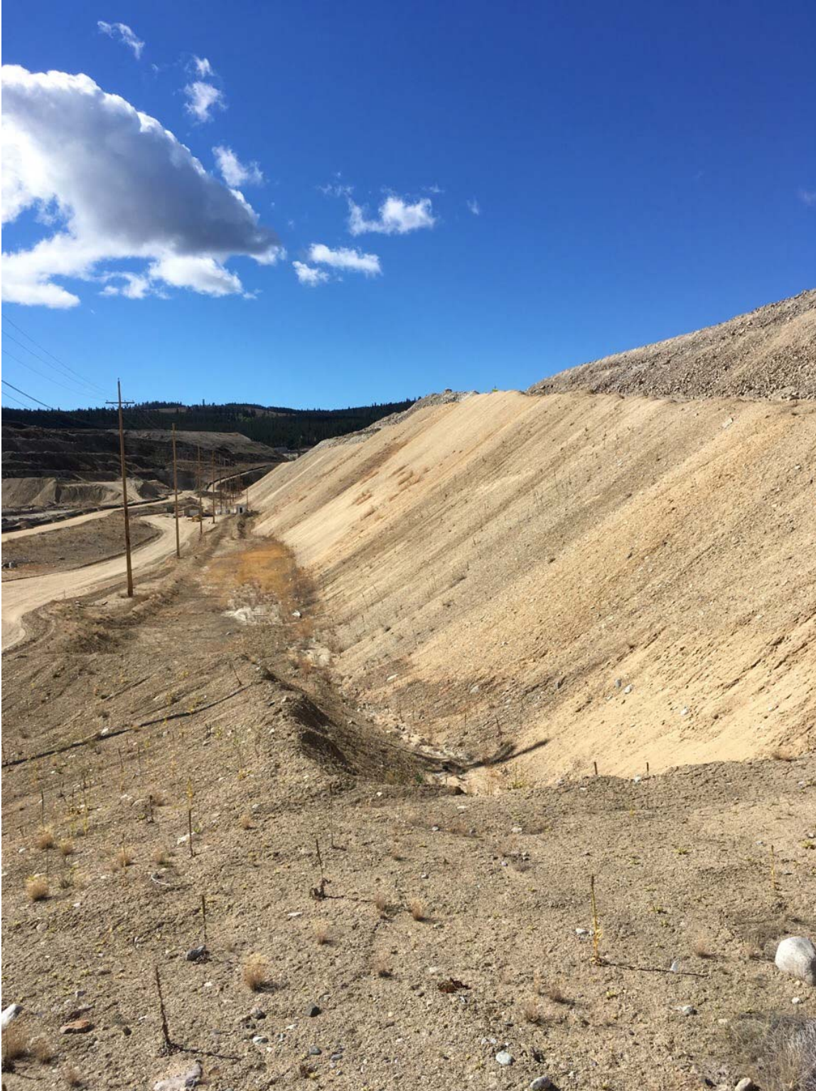
Photo II-B-12 Downstream Toe of Dam - Facing West (HH-2017-13)
