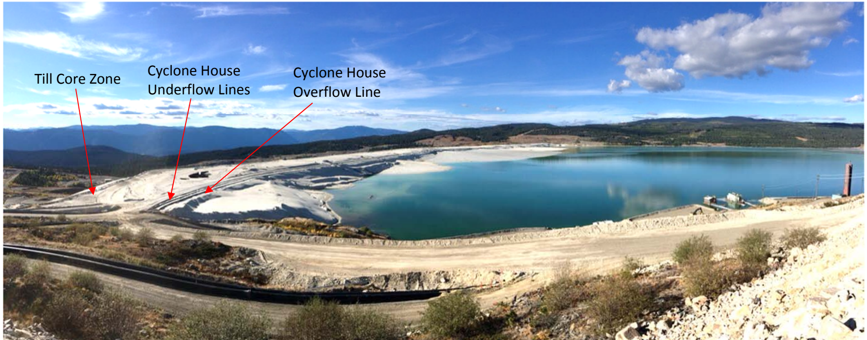
Photo II-A-2 South Abutment Overview (LL-2017-01)
