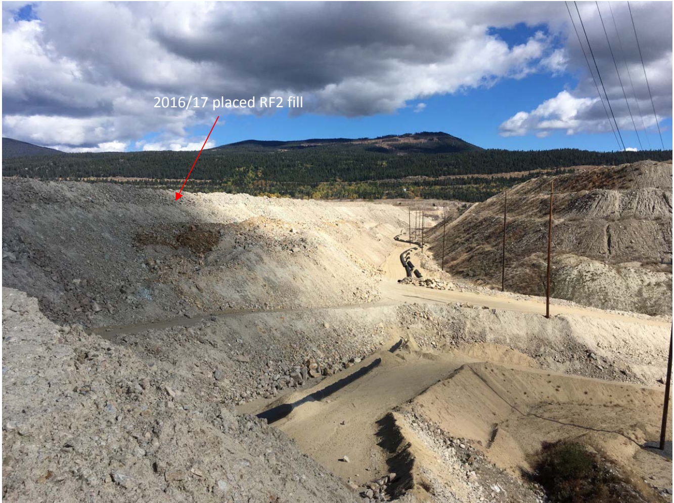
Photo II-B-9 Downstream Face of Dam - Facing Northeast (HH-2017-02)
