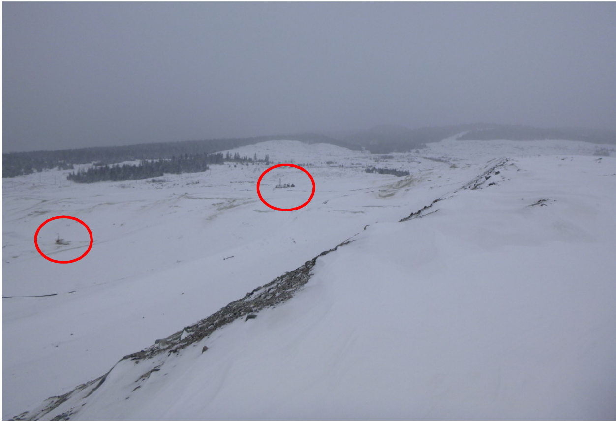
Photo 1- Entire L-L Dam was snow covered at the time of the inspection; two drill rigs seen on the North Buttress Berm (looking North).
