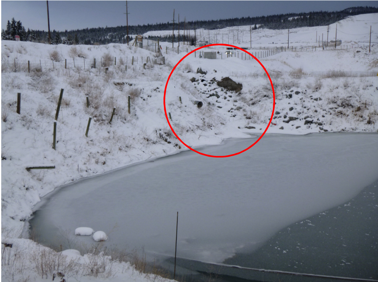
Photo 5 – No flow from Woods Creek Diversion into the Reclaim Pond (looking north).
