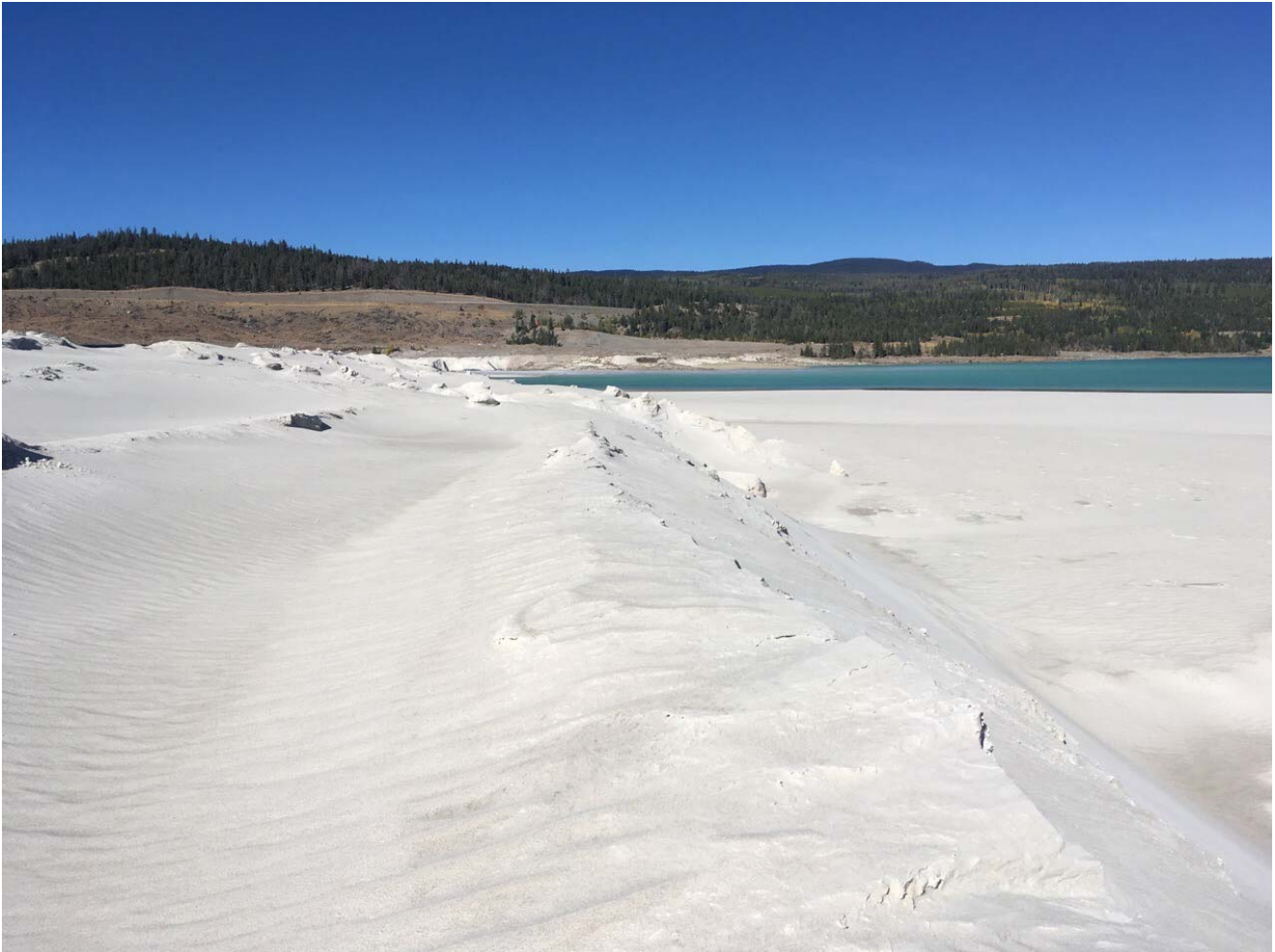
Photo II-A-5 Upstream Dam Face – Beach was Constructed using Hydraulic Sand Panels in 2015 – Facing North (LL-2017-11)
