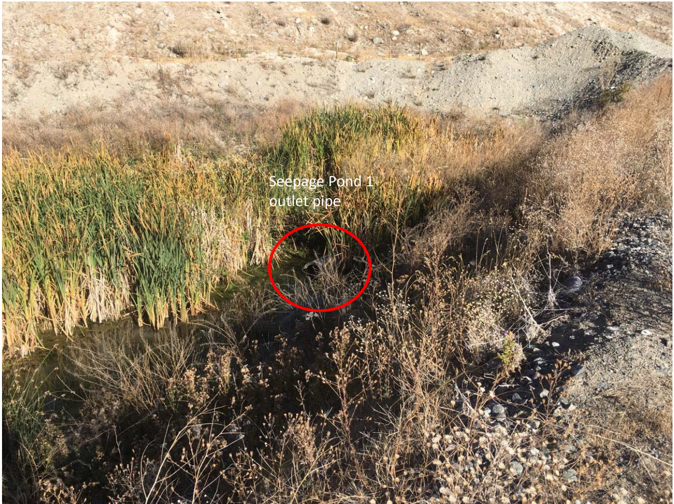
Photo II-C-5 Seepage Pond 1 Outlet (SS-2017-03)
